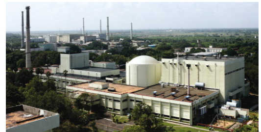
Fast Breeder Test Reactor, Kalpakkam
