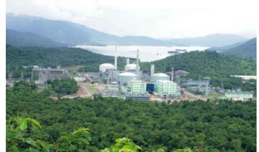
Kaiga Generating Station 1 - 4
