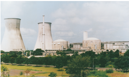
Kakrapar Atomic Power Station Units 1 & 2
